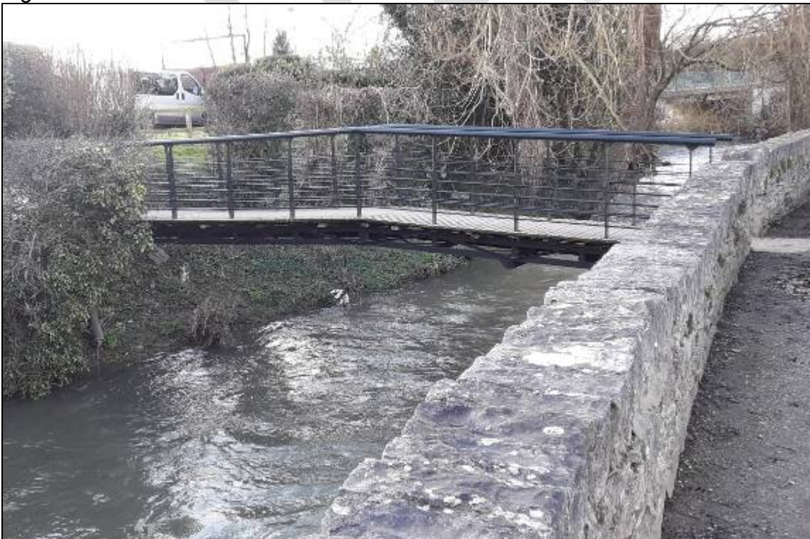
Figure 18: Footbridge over River Ystrad at Brookhouse Mill. Source: NRW
