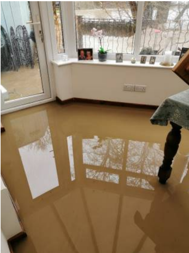
Figure 6: Photo of property ingress of floodwater from Afon Ystrad during Incident at Glan Llyn. Source: Resident
