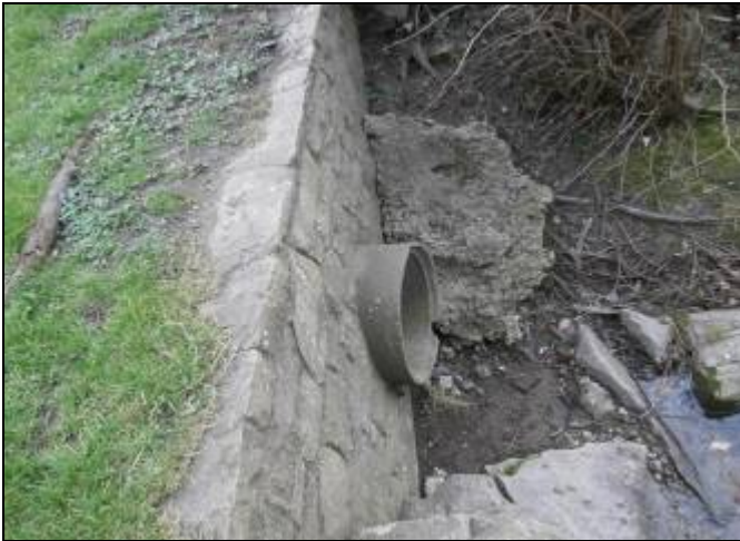
Figure 15 - 400mm Outfall associated with Mill Race Drain
