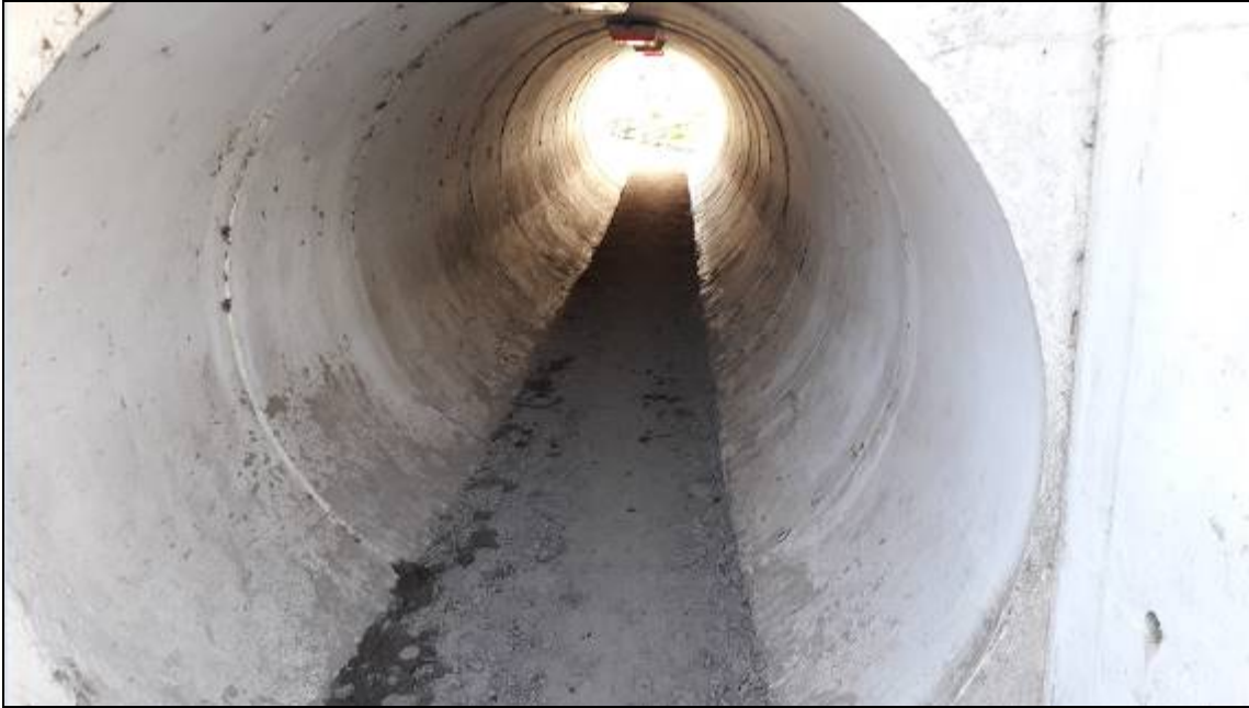
Figure 17: Pedestrian Subway. Source: NRW
