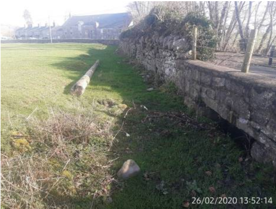
Figure 13 : Photo of Old Mill Outlet. Source NRW
